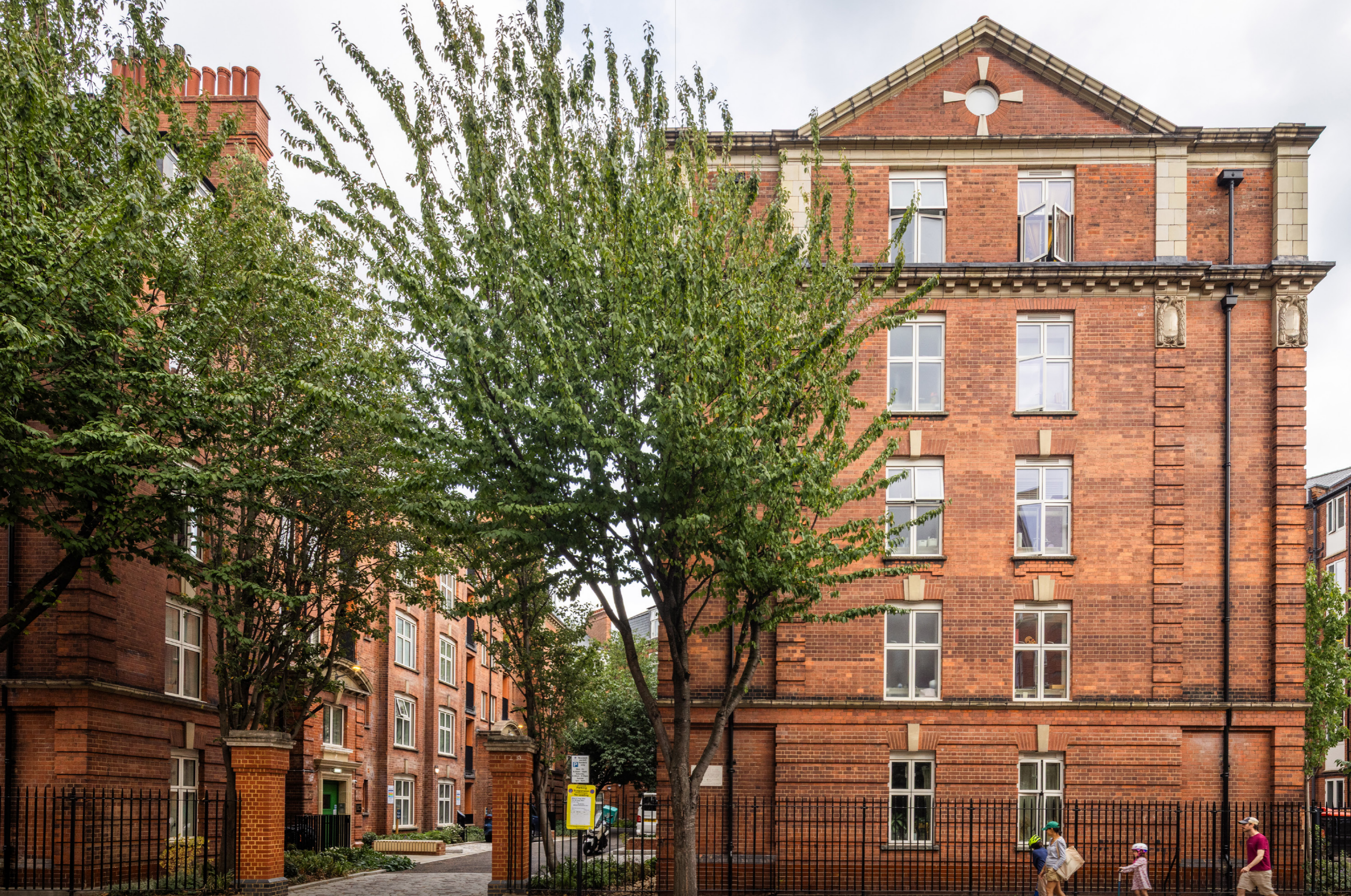
Holistic deep retrofit and landscape transformation for 100 year old Sutton Estate
